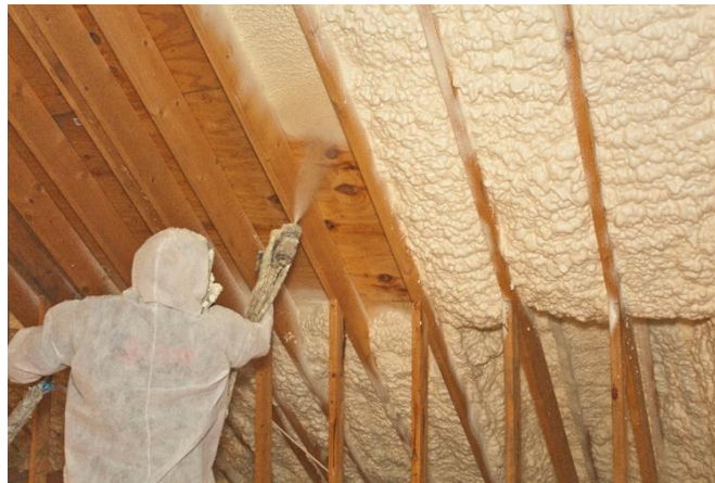
FIGURE 2. APPLICATION OF EASYSEAL.5™ SPRAY FOAM INSULATION IN AN UNVENTED ATTIC
