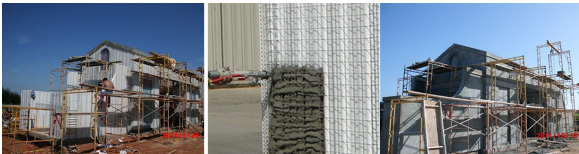
Figure 7. Photos of GCT Insulated Concrete Panels on Site
