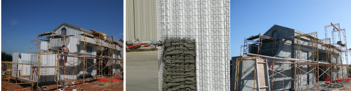
Figure 7. Photos of GCT Insulated Concrete Panels on Site
