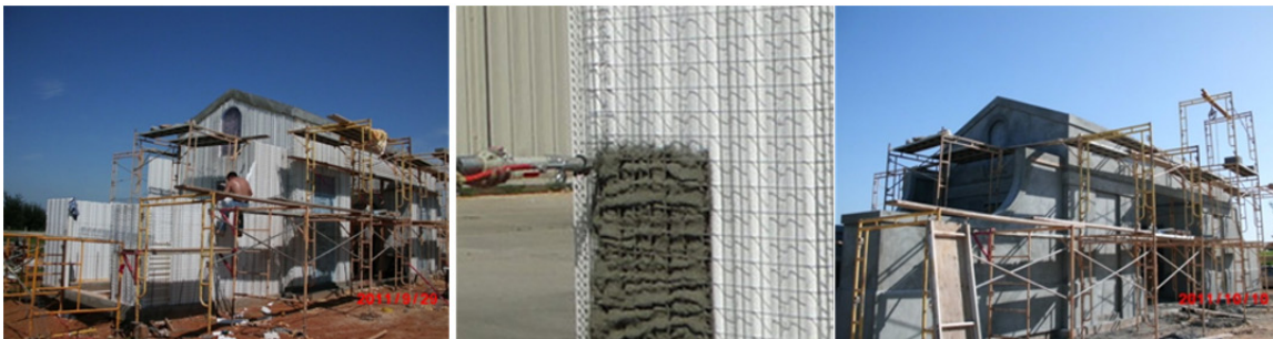
Figure 5. Photos of GCT Insulated Concrete Panels on Site
