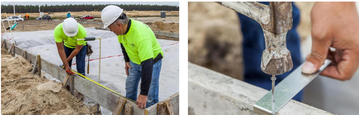
Figure 23. Layout Anchor Brackets and Install Bolts with Proper Spacing
