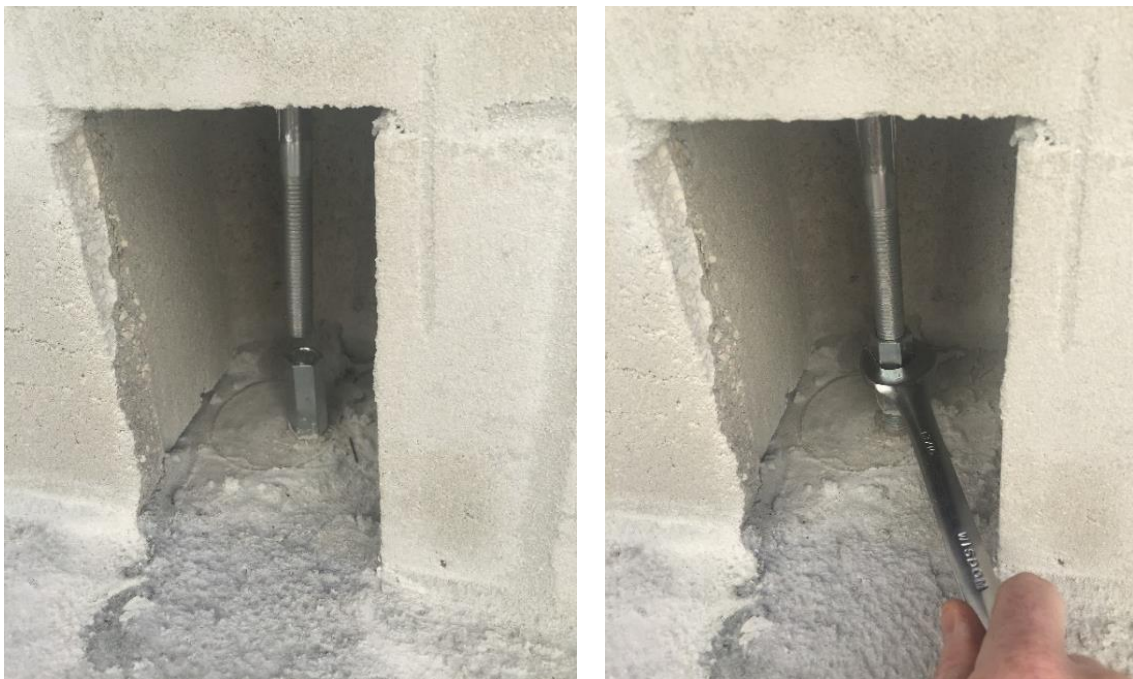
Figure 20. Connecting the Cable to the Anchor Bolt
