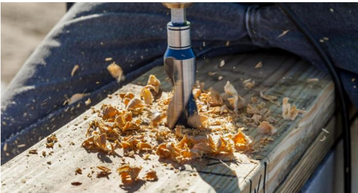
Figure 28. Drill a Hole above each Anchor Bolt
