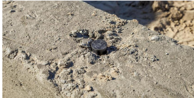
Figure 25. Backing out the Anchor Bolt and Capping the Hole
