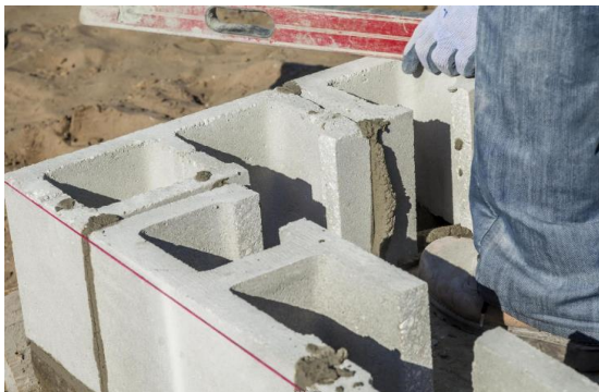
Figure 26. Orient CMU with Openings at Each Cable Location
