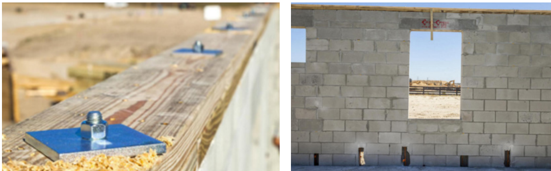
Figure 31. Tighten the Cables Once Epoxy Has Set
