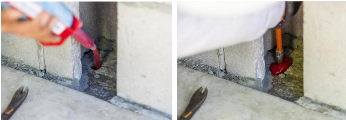
Figure 30. Fill the Anchor Hole with Epoxy
