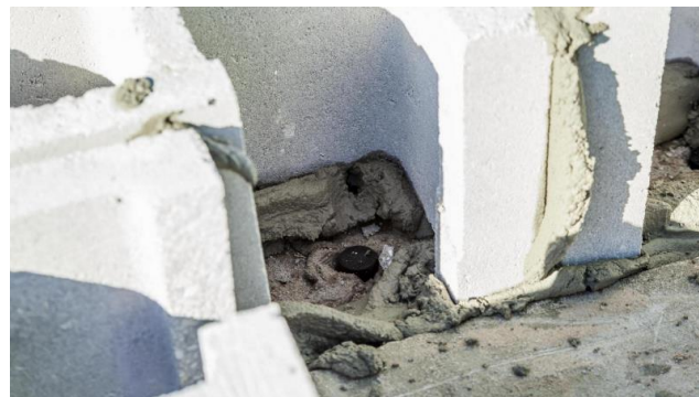
Figure 26. Orient CMU with Openings at Each Cable Location
