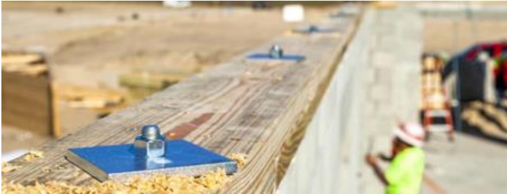
Figure 31. Tighten the Cables once the Epoxy has Set
