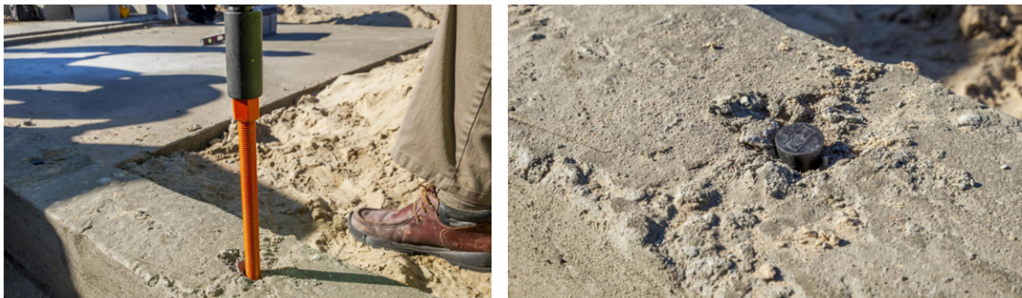
Figure 25. Backing out the Anchor Bolt and Capping the Hole
