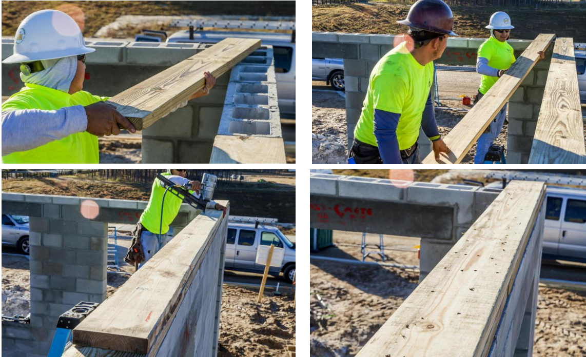
Figure 17. Installation of the Double Top Plate
