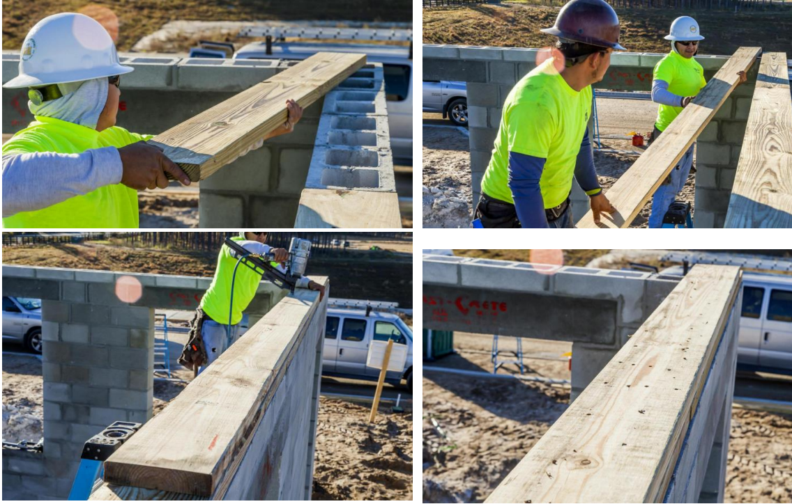
Figure 27. Install Double Top Plate
