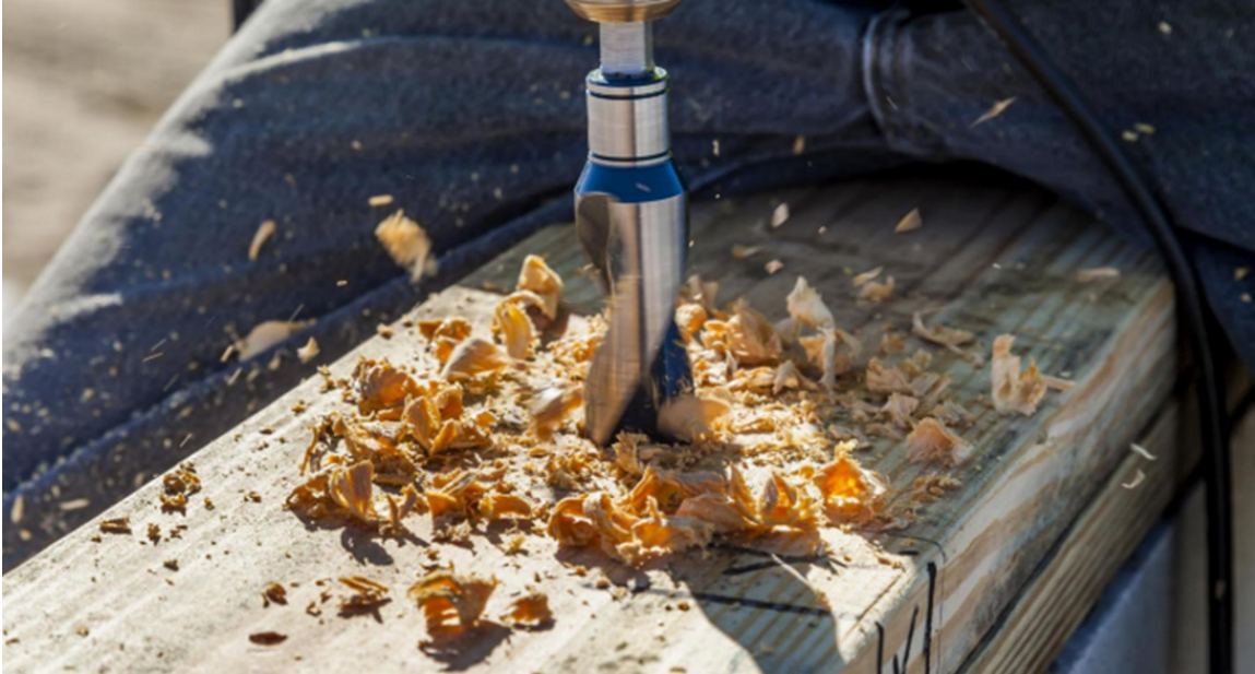
Figure 28. Drill a Hole above each Anchor Bolt
