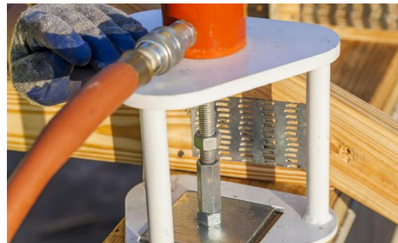
Figure 32. Tension the Cables to the Specified Load
