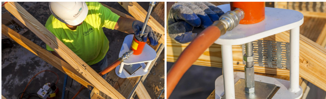
Figure 32. Tension the Cables to the Specified Load
