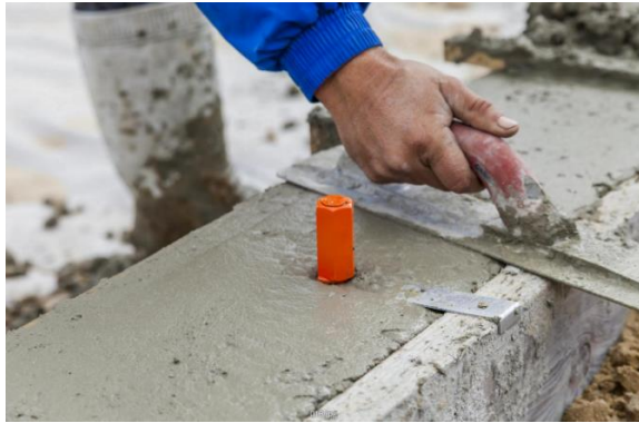
Figure 24. Fill Foundation Forms with Concrete
