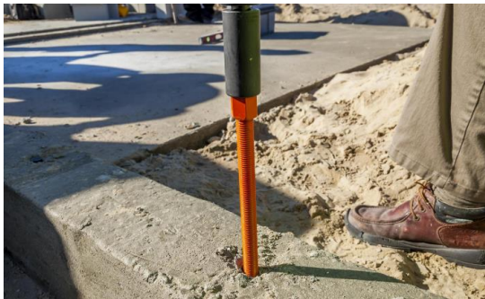
Figure 25. Backing out the Anchor Bolt and Capping the Hole
