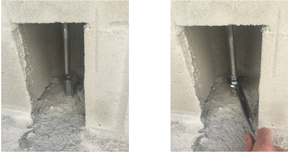
Figure 20. Connecting the Cable to the Anchor Bolt
