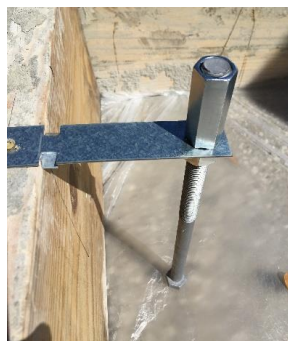
Figure 14. Anchor Bolt Installation
