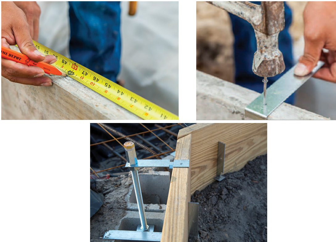
Figure 14. Anchor Bolt Installation
