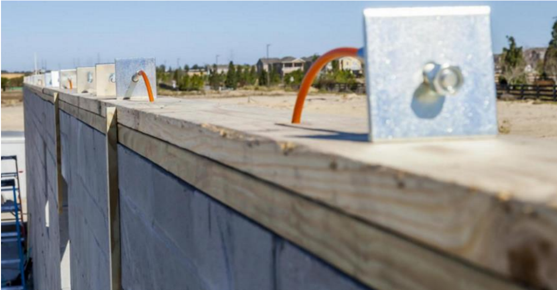
Figure 19. Feed the QTS Cable through the Hole to the Anchor Bolt
