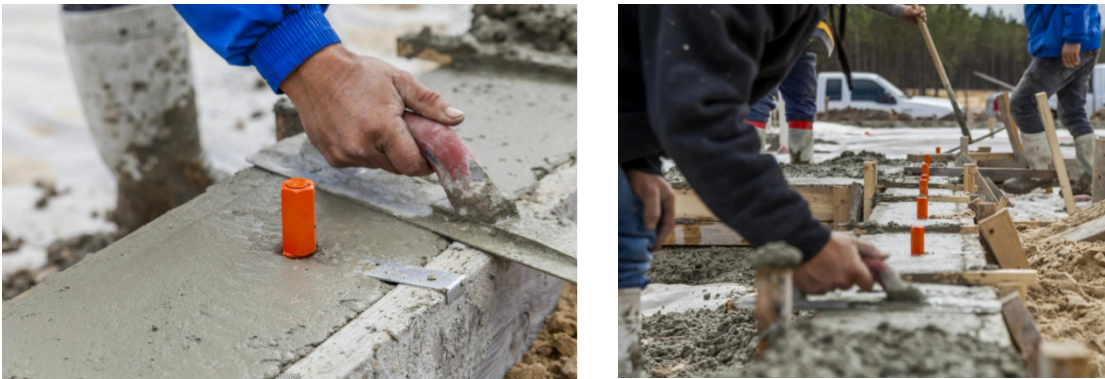
Figure 24. Fill Foundation Forms with Concrete
