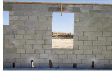
Figure 31. Tighten the Cables once the Epoxy has Set
