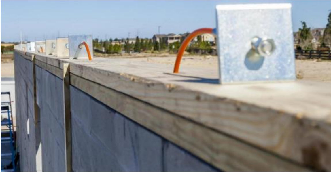
Figure 29. Feed each Cable through the Holes
