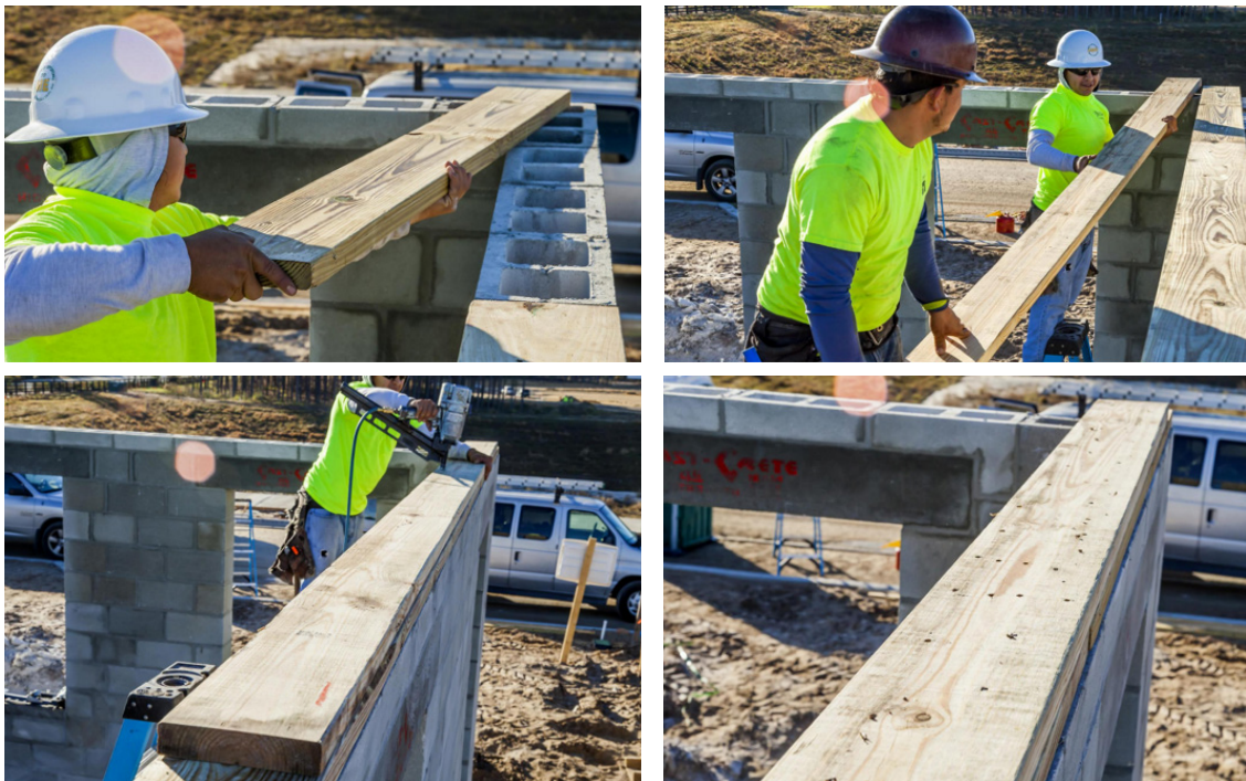
Figure 27. Install Double Top Plate
