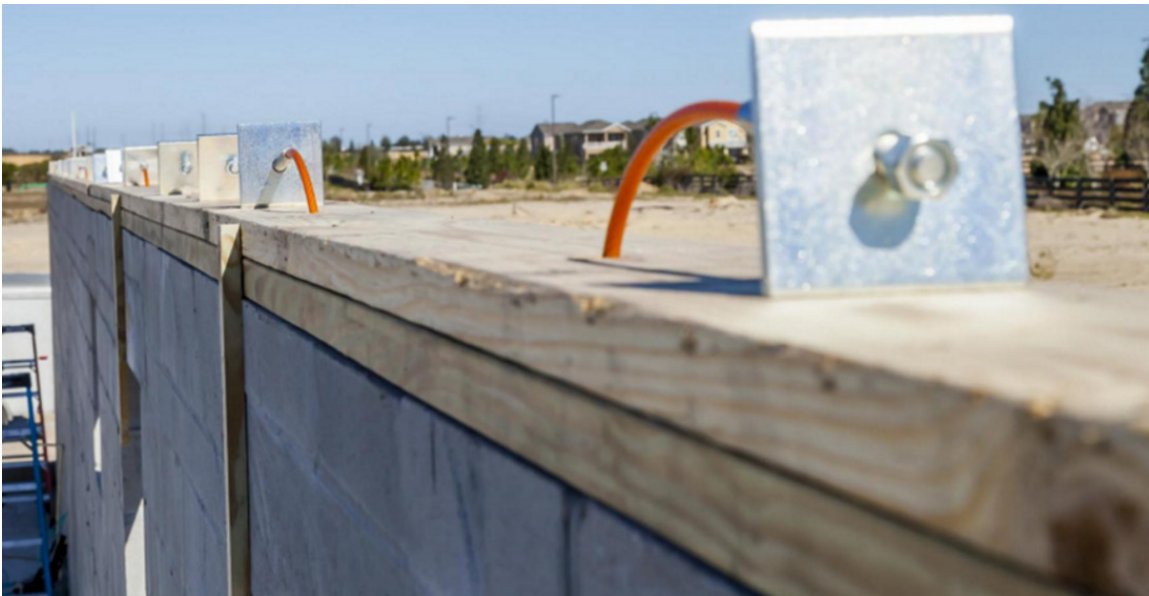
Figure 29. Feed each Cable through the Holes
