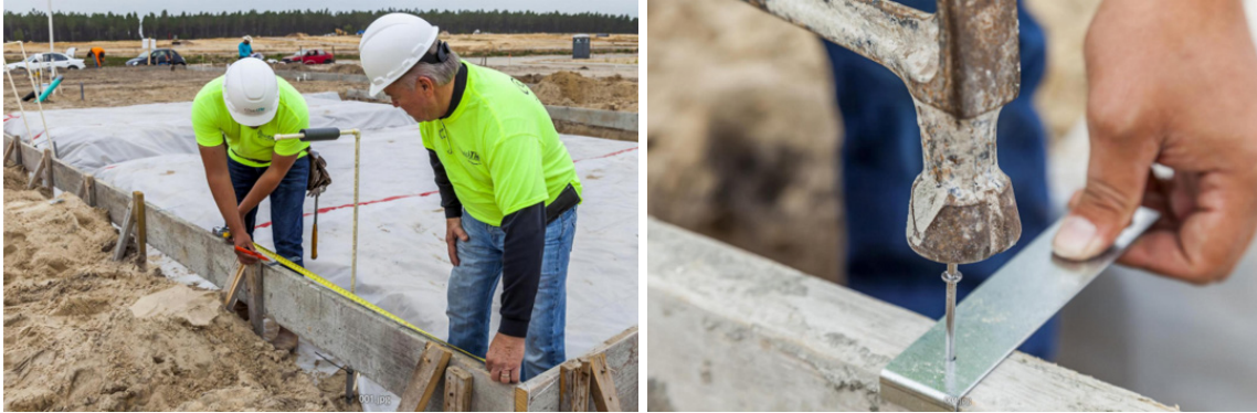
Figure 23. Layout Anchor Brackets and Install Bolts with Proper Spacing
