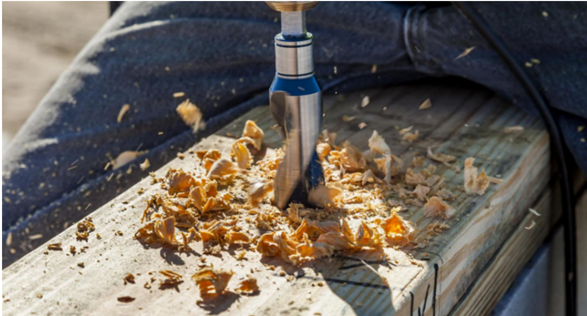
Figure 18. Drill a Hole Above Each Anchor Bolt
