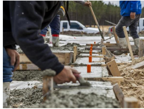
Figure 24. Fill Foundation Forms with Concrete
