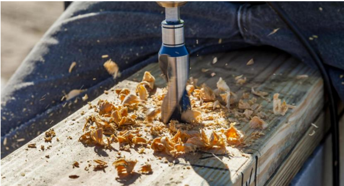
Figure 18. Drill a Hole Above Each Anchor Bolt
