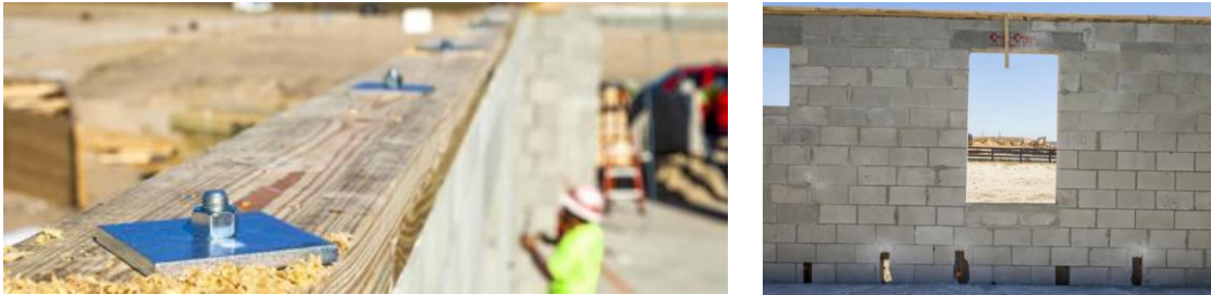
Figure 21. Tighten the Bolt on the Top Plate to Remove the Slack from the Cable
