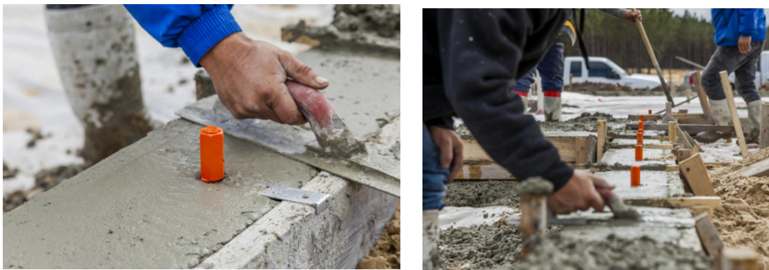
Figure 15. Fill Foundation Forms Around the Anchor Bolts
