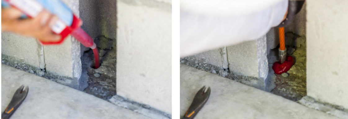
Figure 30. Fill the Anchor Hole with Epoxy
