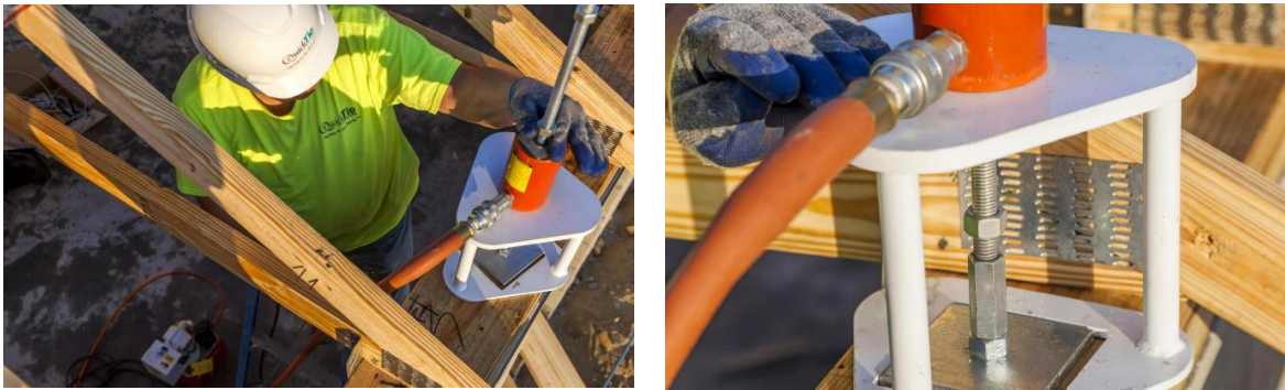
Figure 22. Tension the Cables to the Specified Load
