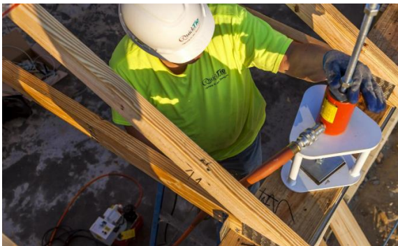
Figure 32. Tension the Cables to the Specified Load
