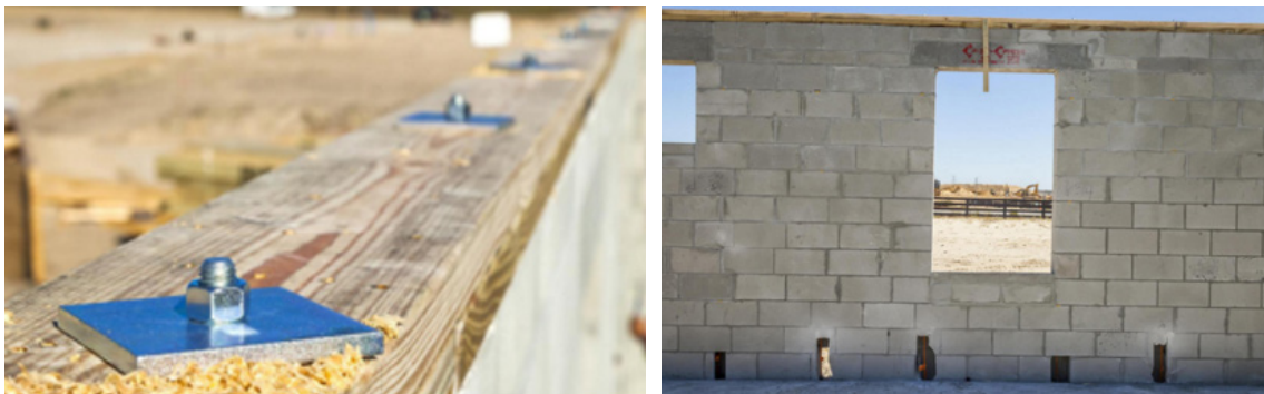
Figure 21. Tighten the Bolt on the Top Plate to Remove the Slack from the Cable
