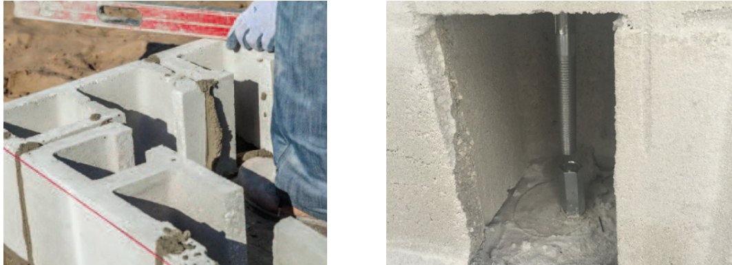
Figure 16. Place CMU with Openings at QuickTie Anchor Bolt Locations
