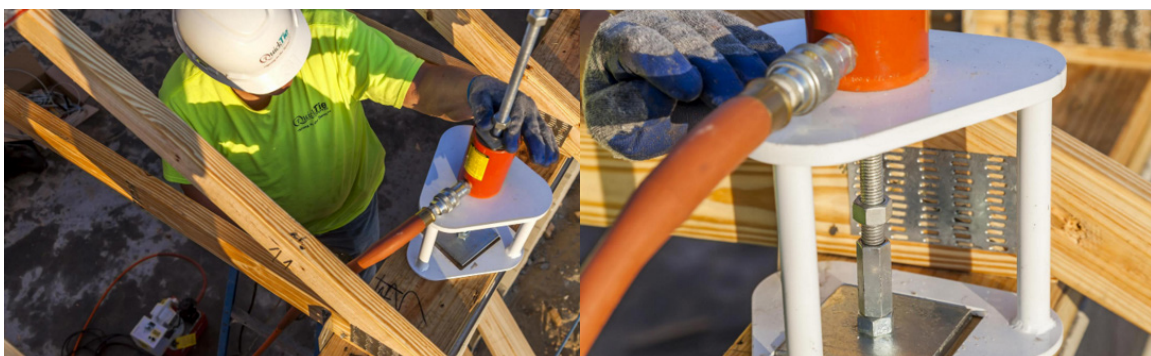
Figure 22. Tension the Cables to the Specified Load
