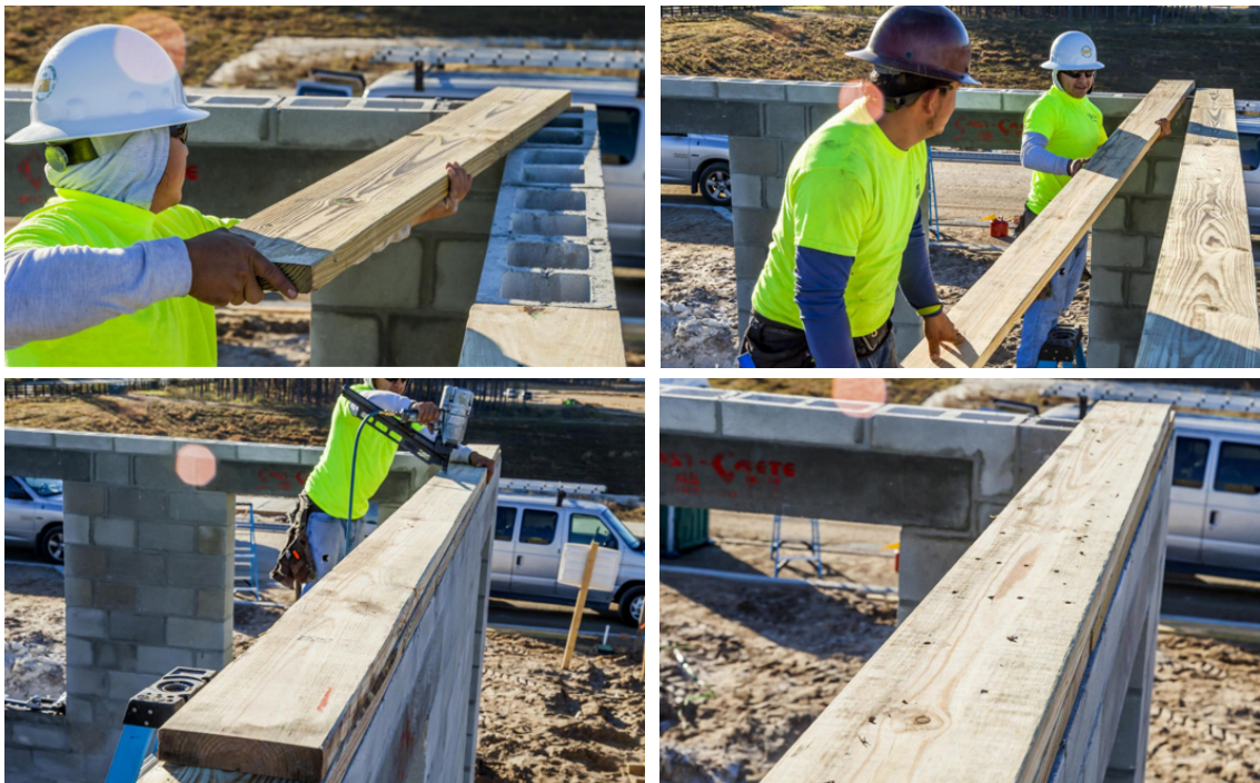
Figure 17. Installation of the Double Top Plate
