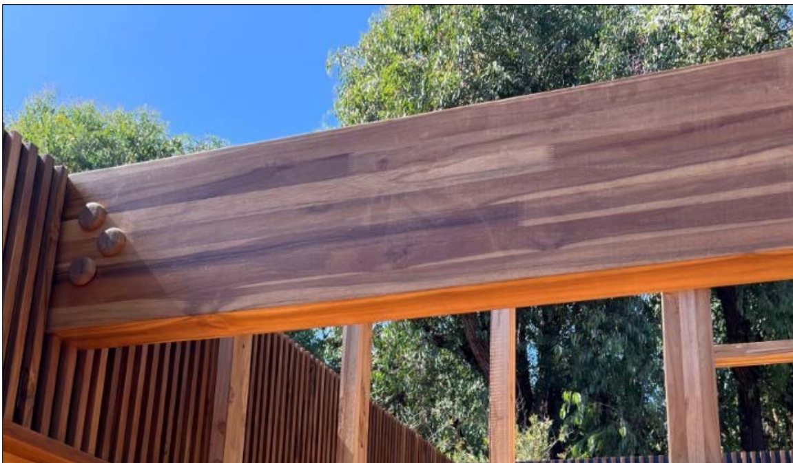
Figure 1. Masaya Teak Glued Laminated Timber
