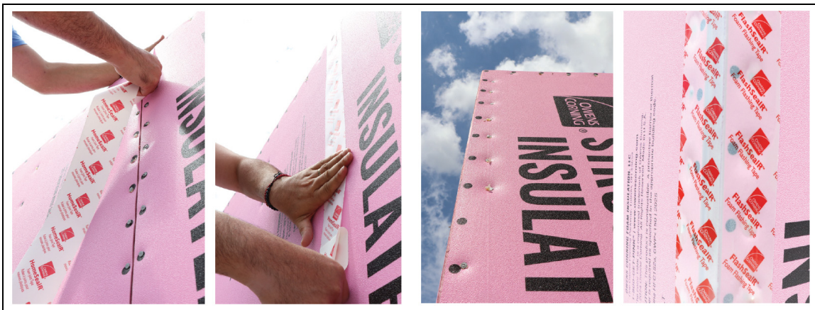
Figure 7. Typical Seam Flashing Detail
