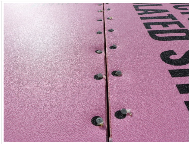
Figure 4. Fastening Indentation Example
