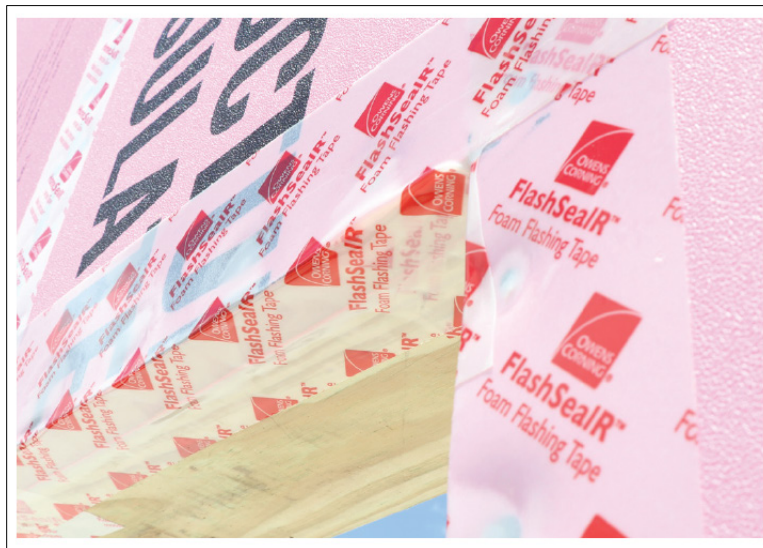
Figure 9. Typical Window Flashing Detail
