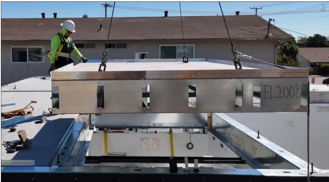
Figure 1. Installation of Shera Board Diaphragm Panel
