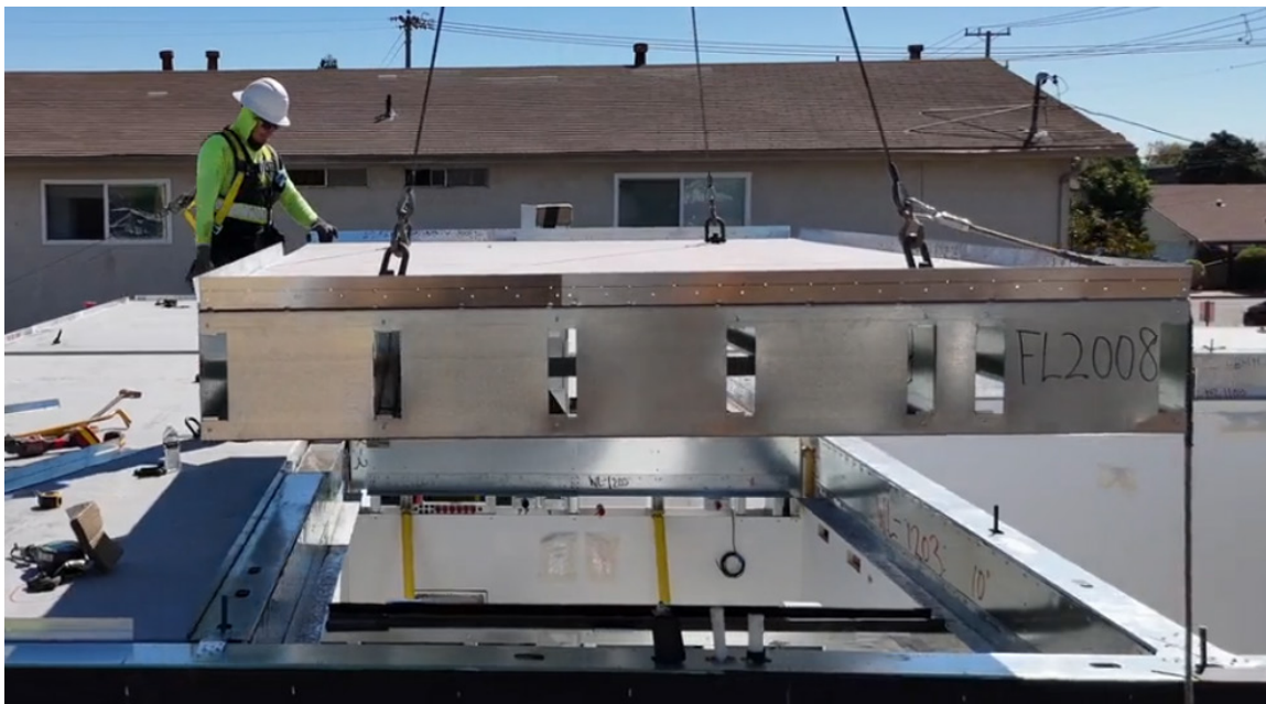
Figure 1. Installation of Shera Board Diaphragm Panel
