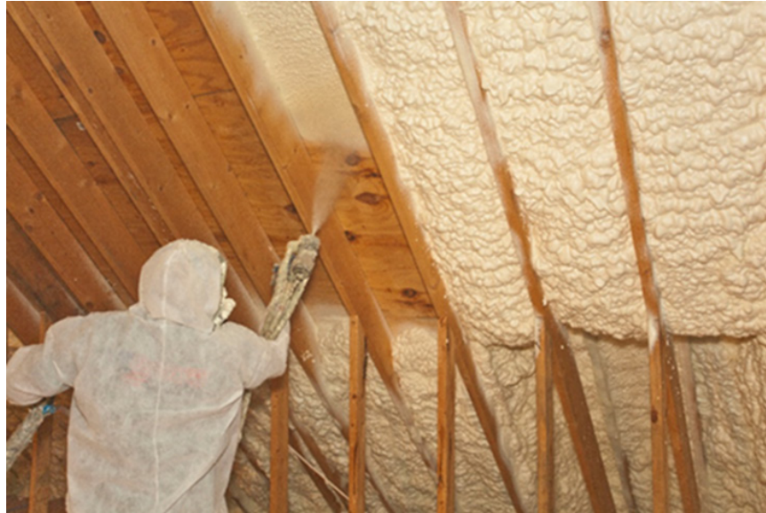
Figure 2. Application of Enverge EZ-U Spray Foam Insulation in an Unvented Attic
