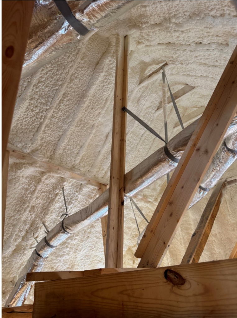
Figure 2. Application of Enverge EZ-U Spray Foam Insulation in an Unvented Attic
