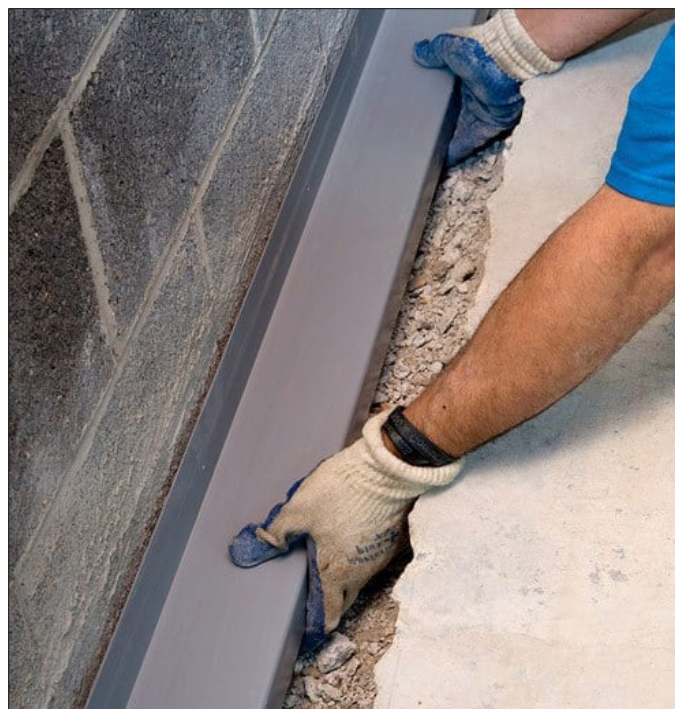
Figure 3. WaterGuard and WaterGuard XL Sub-Floor Drainage Systems – Typical Installed Location
