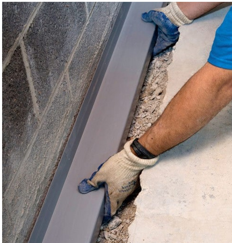
Figure 3. WaterGuard Sub-Floor Drainage System - Typical Installed Location
