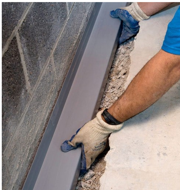
Figure 3. WaterGuard Sub-Floor Drainage System - Typical Installed Location
