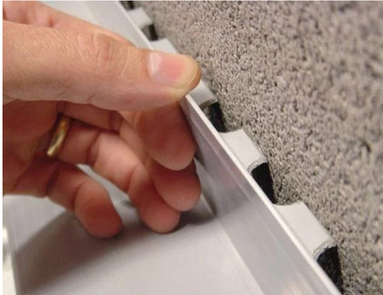
Figure 5. WaterGuard Sub-Floor Drainage System – Conduit
