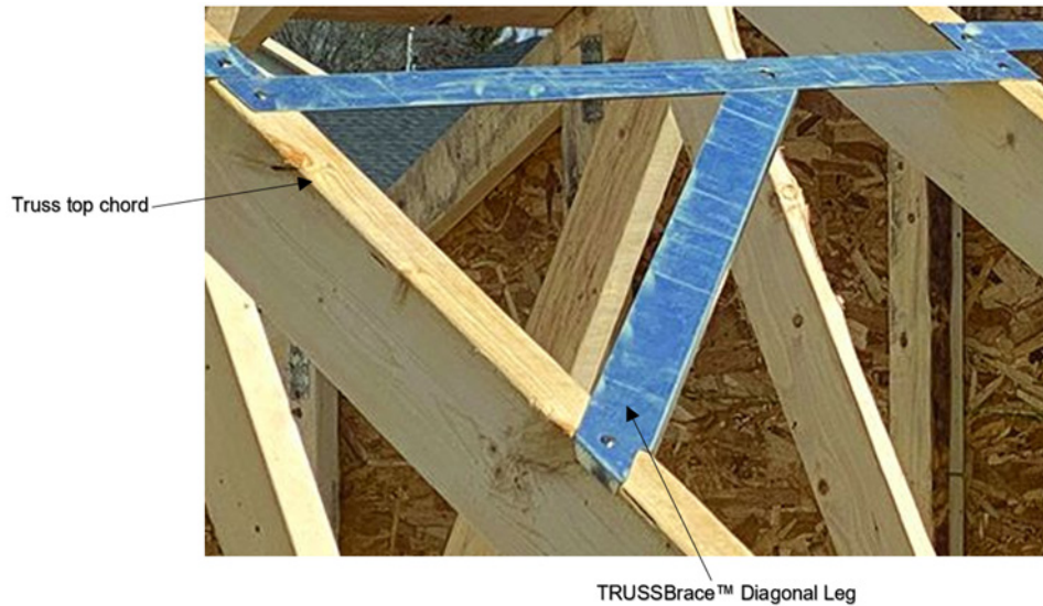
Figure 3. TrussBRACE Connection to Truss Top Chord
