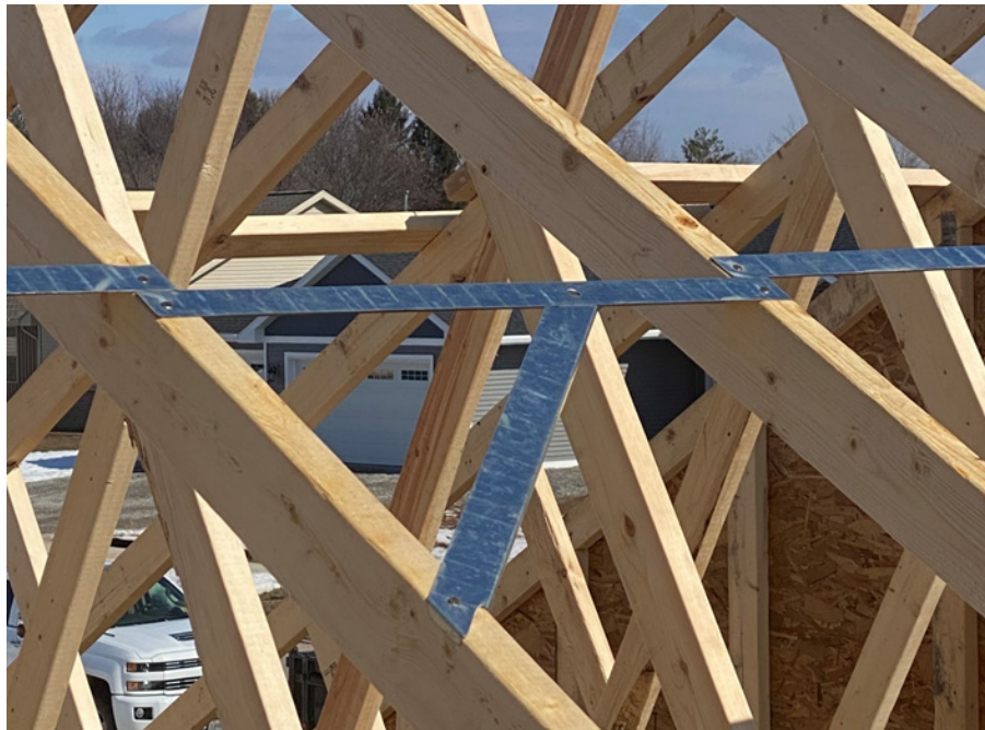
Figure 1. FastenMaster TrussBRACE Installed on Truss Top Chords
