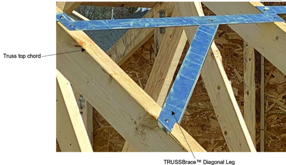
Figure 3. TrussBRACE Connection to Truss Top Chord
