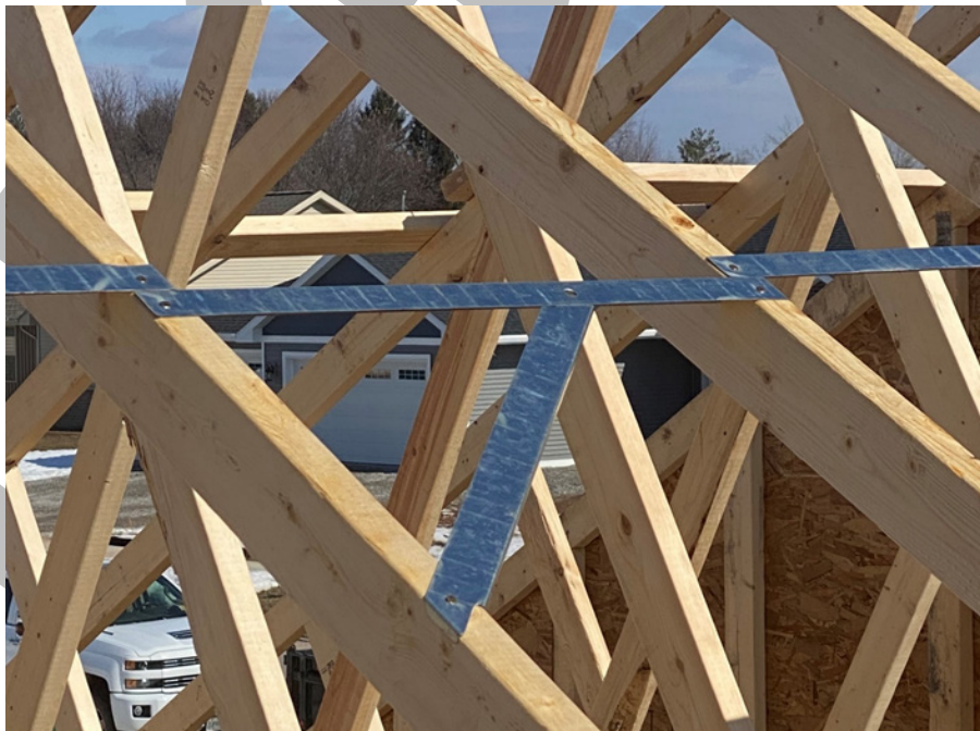
Figure 1. FastenMaster TrussBRACE Installed on Truss Top Chords
