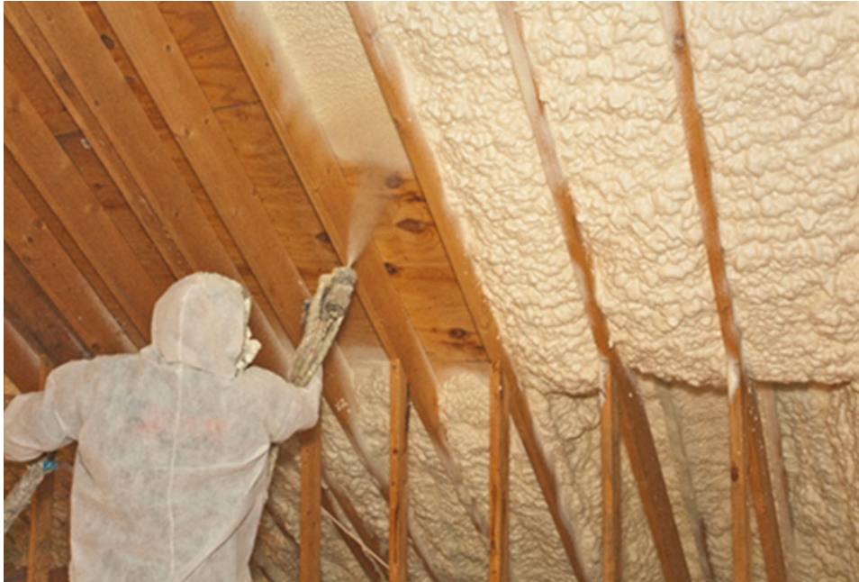
Figure 2. Application of Enverge EasySeal .5 Spray Foam Insulation in an Unvented Attic
