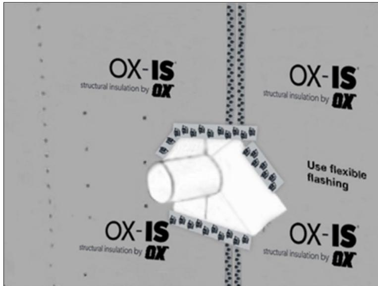
Figure 5. Typical Penetration Flashing Detail – Unflanged
