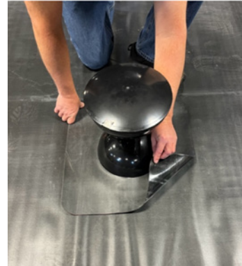
Skirt on the VacuSeal Vent Secured Roofing System is Adhered Using Double-Sided Butyl Tape or hot air welded, depending on the skirt material, to the Roofing Membrane
