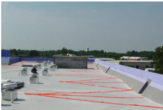
Distribution Strips Connect the Roof Perimeter to the VacuSeal Vent Secured Roofing System
