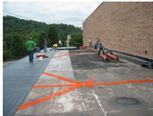
Roof Membrane is Placed Over the Distribution Strips
