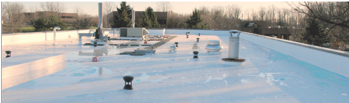
Position of VacuSeal Vent Secured Roofing Systems are Staggered to Accommodate Variations in Wind Speed on a Completed Roof Application
