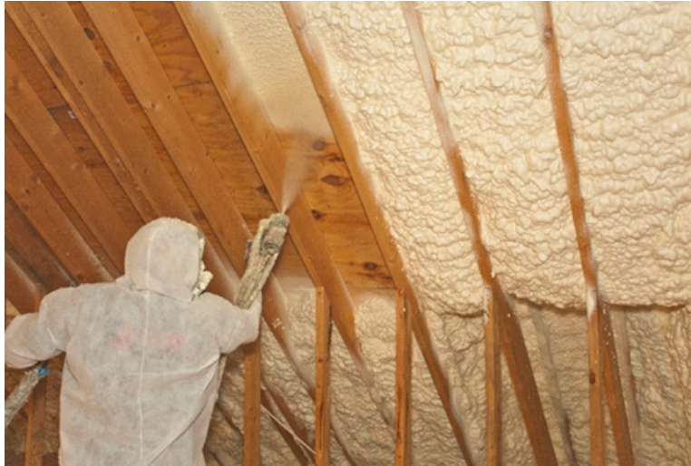
Figure 2. Application of EasySeal ULD Spray Foam Insulation in an Unvented Attic
